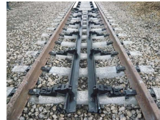
Turned over rails for track maintenance work
